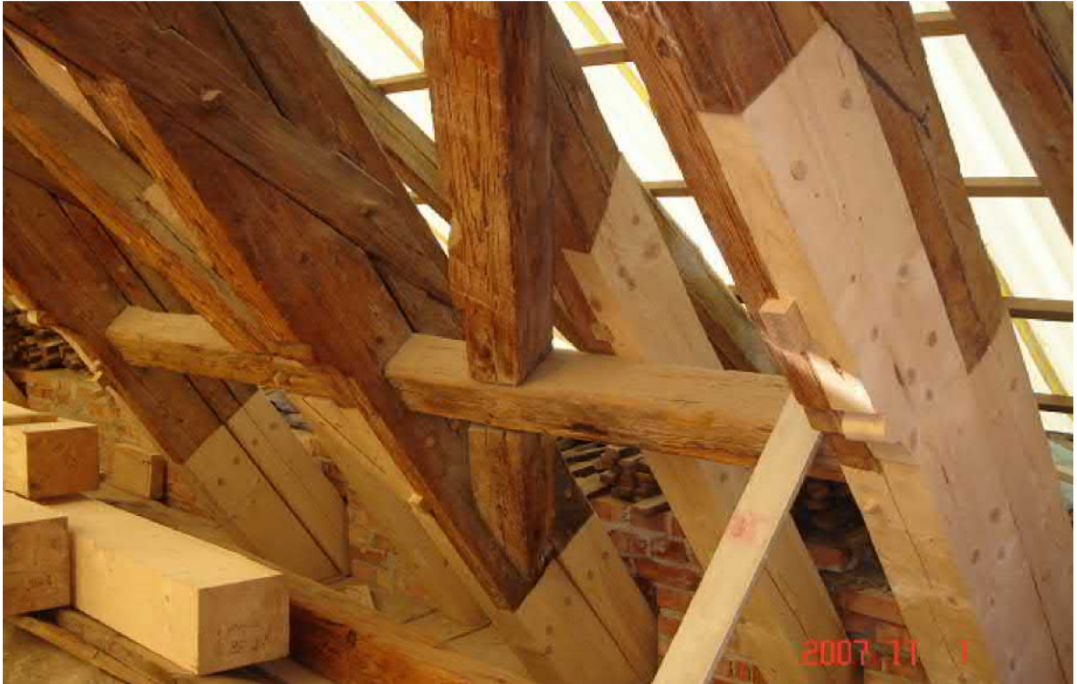
Figure 48. Timber prosthesis with all-timber connections used similarly as could be applied to rafters and posts in Louhisaari manor. This intervention method has been used in a building located in Prague. [22, p. 69]
