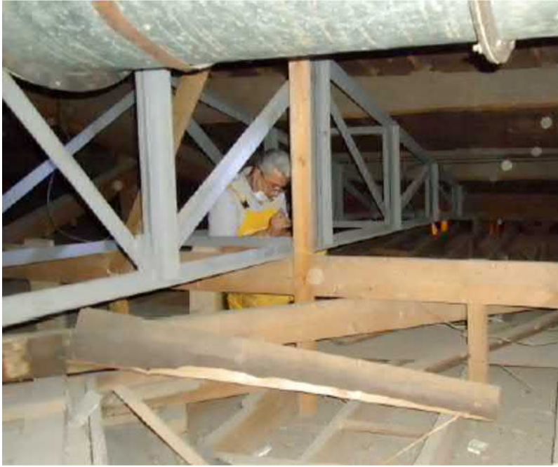
Figure 15. Additional steel roof trusses are installed to increase the load-bearing capacity of the timber roof structures [49, p. 5].
